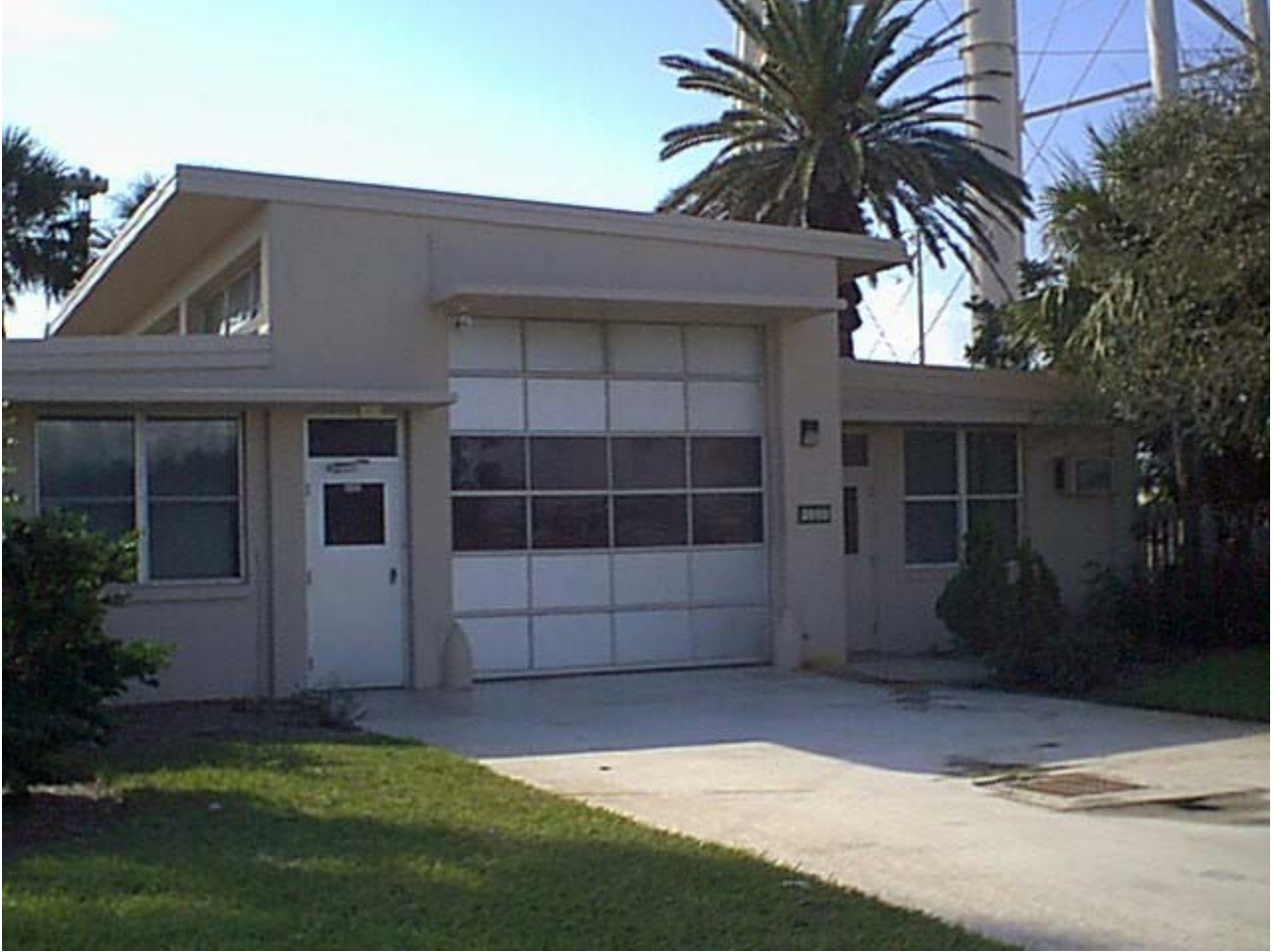
FIGURE 1 – SOUTH HOUSING FIRE STATION, 12/27/00
