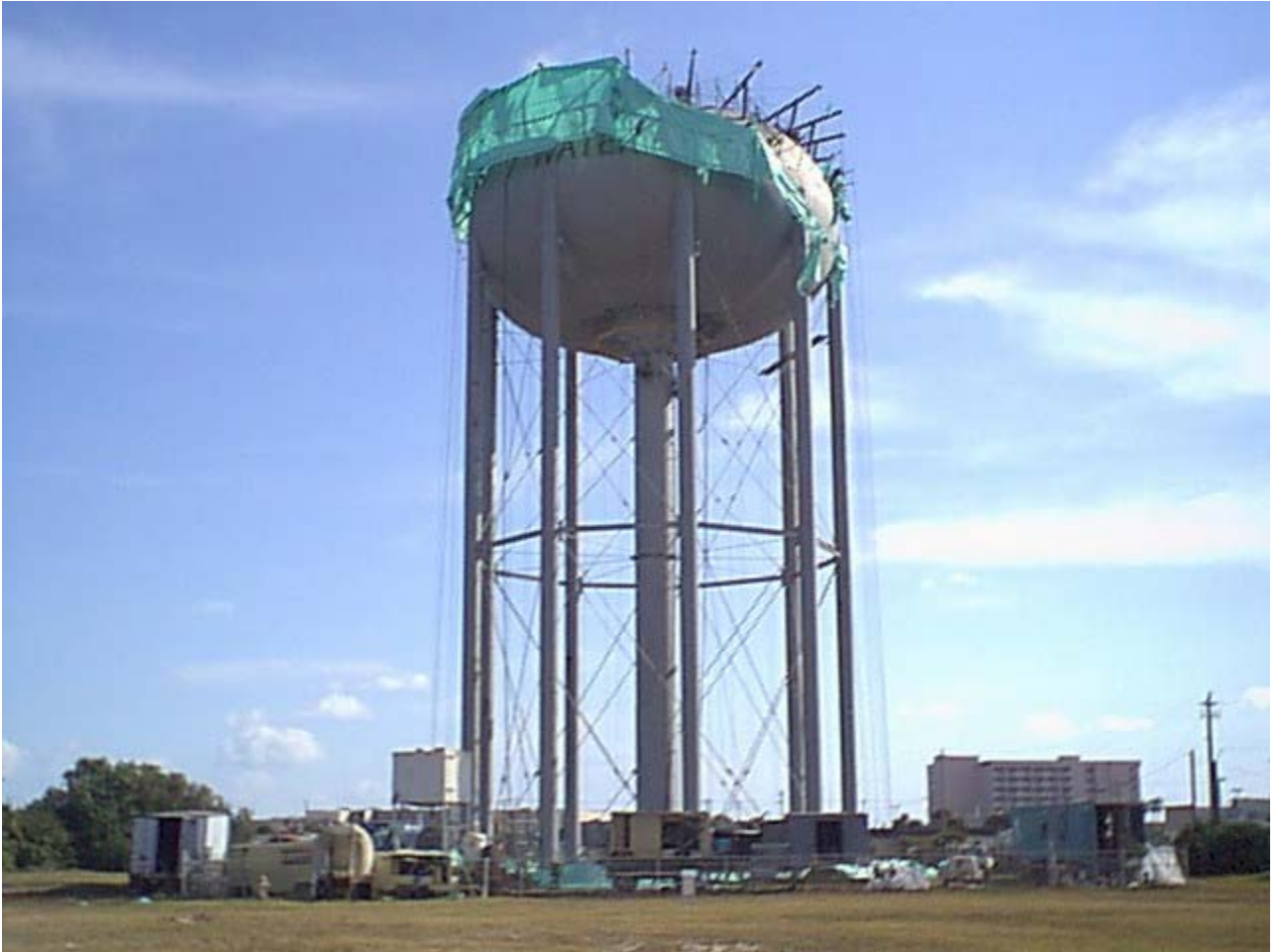
FIGURE 1 - SOUTH HOUSING ELEVATED WATER STORAGE TANK, WITH CONTAINMENT TARP, 12/27/00
